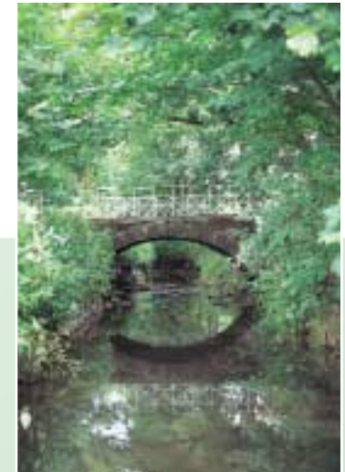
Iron Bridge, River Alt, Croxteth Park
